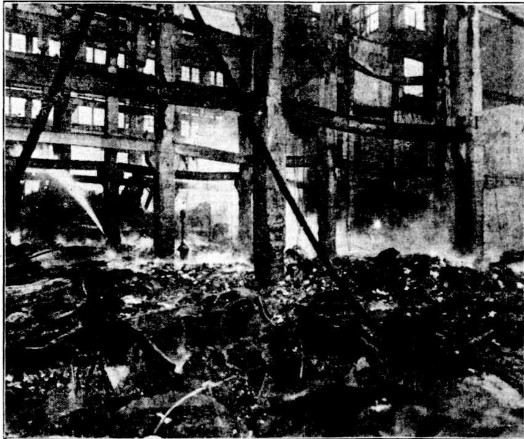
A comprehensive idea is here conveyed of the appearance of the interior of Richards' Buildings on Tuesday morning. The rolled steel I beams between the columns were buckled and twisted, indicating the phenomenal heat generated by the blaze. The completeness of the havoc and ruin wrought by the fire is also graphically illustrated.
