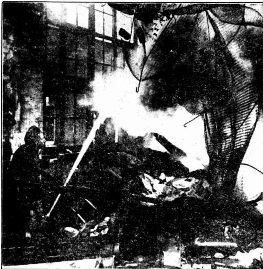
HEEDLESS OF FALLING RUINS FIREMAN OPERATES AMONG TWISTED MOTOR CHASSIS.
