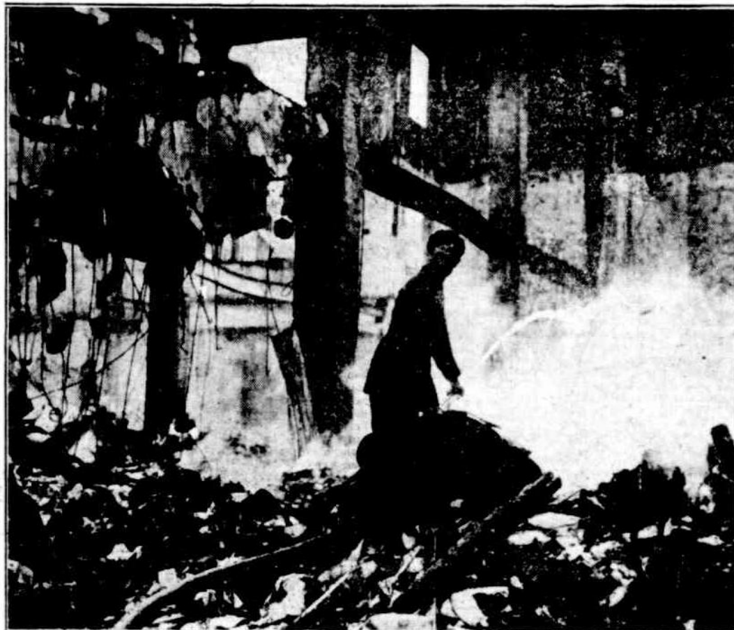
Fireman playing a powerful water jet on to the smouldering debris. The photo incidentally gives a vivid idea of the outer shell and the columns, the sole remaining evidences of the handsome construction that was once Richards Buildings.
